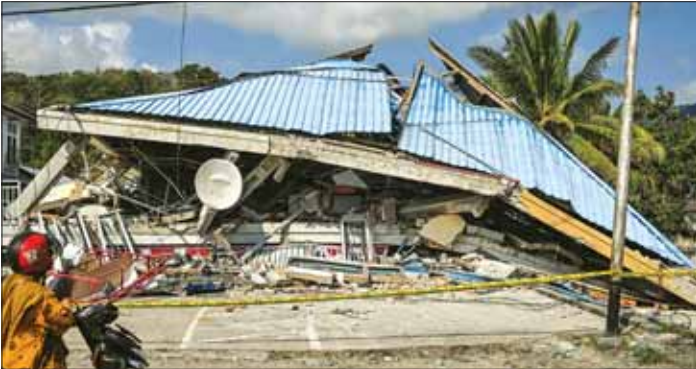
A collapsed building following a 7.7-magnitude earthquake in Borong, East Manggarai, East Nusa Tenggara, yesterday. (AFP)
