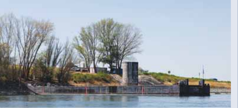
A barge is in place for the potential sinking to raise the Danube's water level near the Paks Nuclear Power Plant in Dunaszentbenedek, Hungary. (Reuters)
