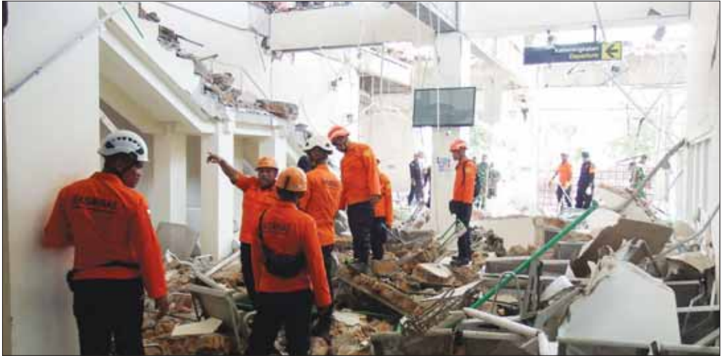
Rescuers inspect a heavily-damaged building at L Say port following an earthquake in Maumere, Sikka, East Nusa Tenggara province, Indonesia, yesterday. (Reuters)
